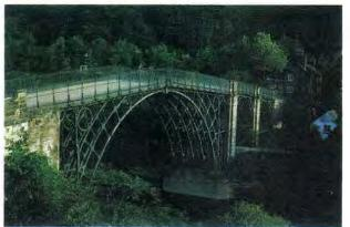
**Figure 14.9:** The bridge at Ironbridge was the first ever bridge built of iron and was awarded UNESCO World Heritage status in 1986. It has a span of around 30m.
