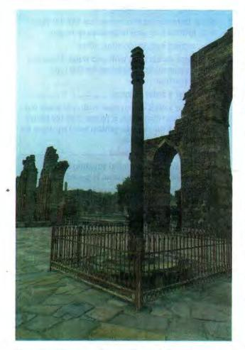
**Figure 14.8:** The Iron Pillar of Delhi dates from the beginning of the 5th century and is remarkable for its resistance to rusting.
