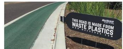
▲ Figure 19.42 Plasphalt is made up of grains of plastic produced from unsorted plastic waste. This replaces the sand and gravel usually used in asphalt production for road surfaces. It can also contain recycled glass pellets
