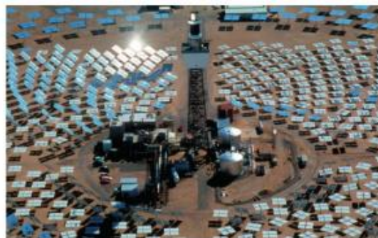
▲ Figure 17.16 A large number of mirrors focus heat from the Sun on a boiler in the tower at the centre. The steam produced drives a turbine to generate electricity.
