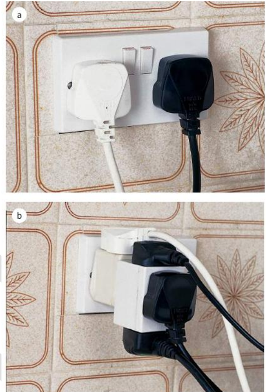
Figure 10.19 a Correct use of an electrical socket. b Here, too many appliances (resistances) are connected in parallel. This reduces the total resistance and increases the current drawn, to the point where it becomes dangerous.
