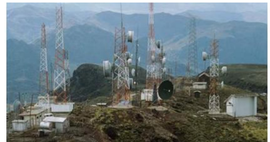
Figure 13.13 These telecommunications masts are situated 4500 metres above sea level in Ecuador. They transmit microwaves, a form of electromagnetic radiation, across the mountain range of the Andes.
