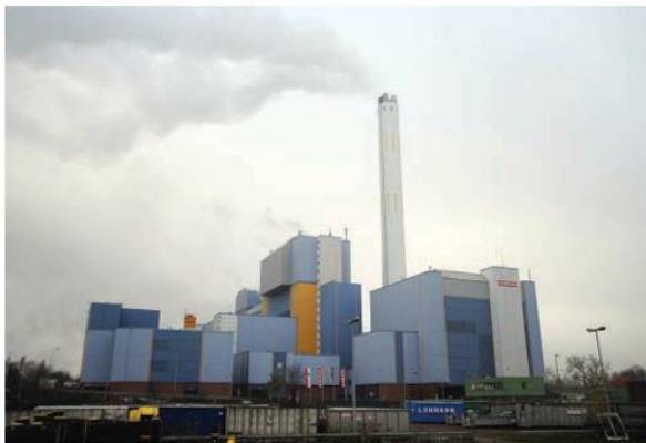
▲ Figure 12.22 Incineration plants can burn waste material to produce heat which can be used to provide warm water or can be converted into electricity
