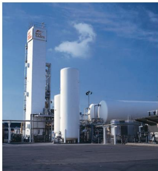
▲ Figure 14.19 Gases from the air are extracted in this fractional distillation plant
