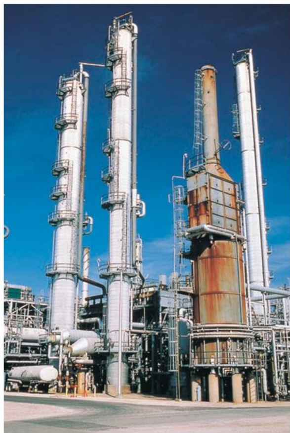
a Fractional distillation of petroleum in a refinery
