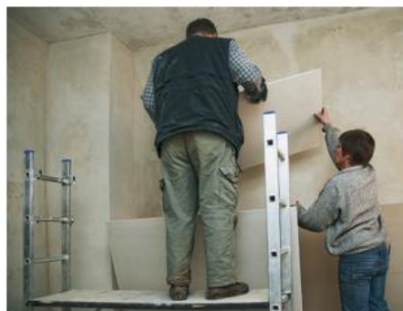
▲ Figure 11.20 This plasterboard is made using calcium sulfate from an FGD plant
