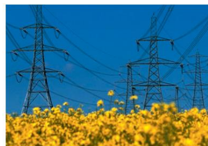
b Due to the high density of copper and its cost, steel-cored aluminium cables are used for electrical transmission through national grids
