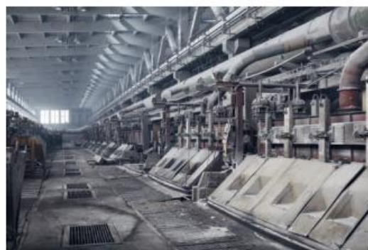
▲ Figure 5.7 An aluminium smelting plant
